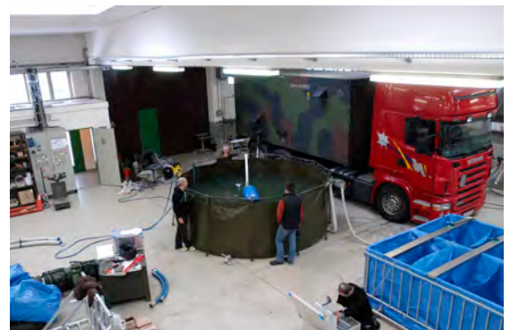
Water purification plant for decontamination purpose; technical test set-up
