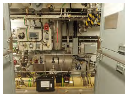
Examination of the pollutant load in operating rooms on marine ships (F125)
