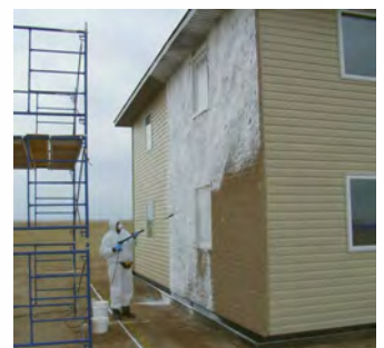
Decontamination of infrastructure
