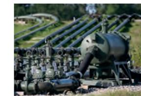
The special infrastructure pipeline training facility is the only of its kind in Europe filled with real fuels. This enables trainees to apply and practice their skills under live conditions. Training is conducted on modular bulk fuel installations with capacities ranging from 150 m<sup>3</sup> to 1,200 m<sup>3</sup>, sections of static pipeline systems, and the associated mobile back-up systems.
